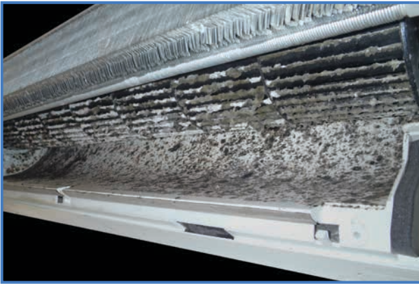
Mini-Split blower with MOLD
